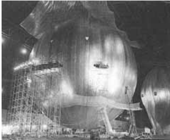
Echo II passive communications satellite undergoes pre-flight inflation tests.
